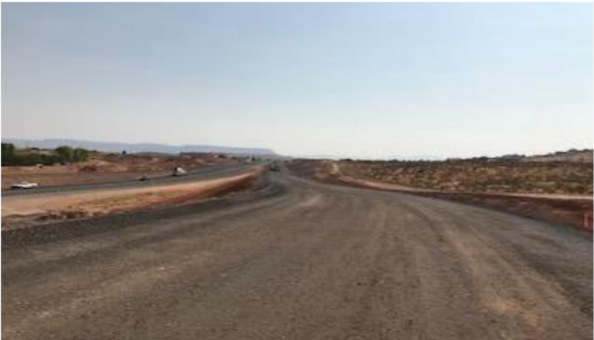
Placement of Untreated Base at the SR-9 off-ramp
