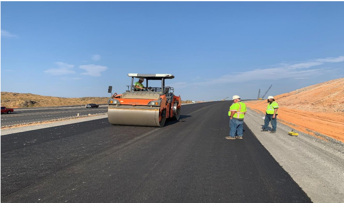
Asphalt placement on the new on-ramps and off-ramps
