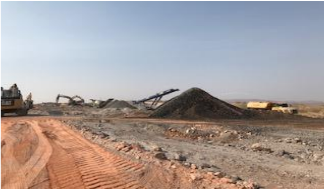
Onsite Crushing Operation
