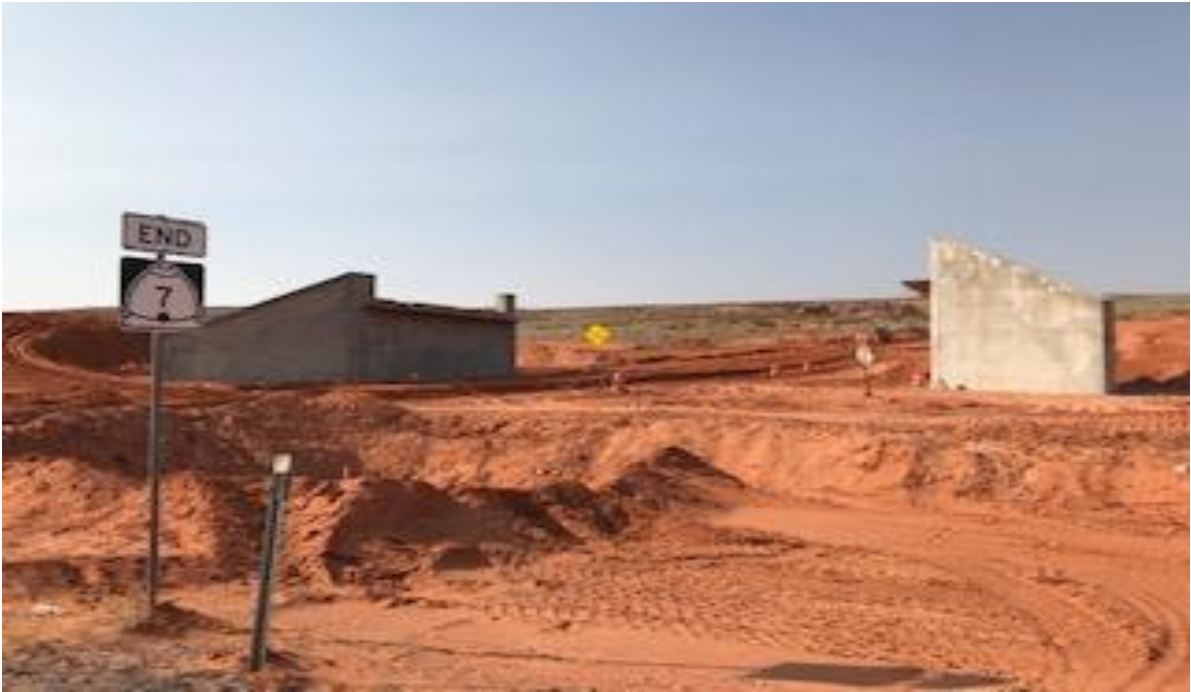
Construction of future overpass at 4300 West
