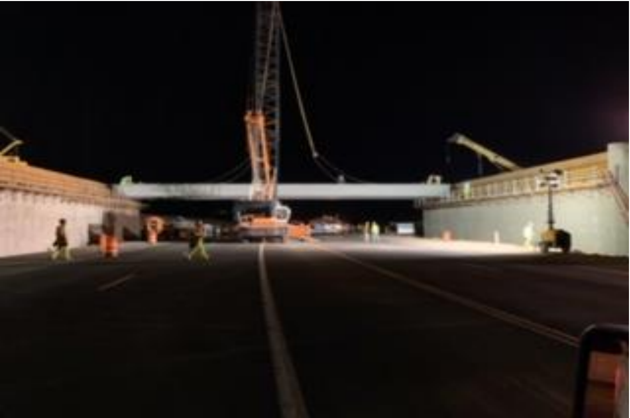
Girder placement at the new SR-9 overpass
