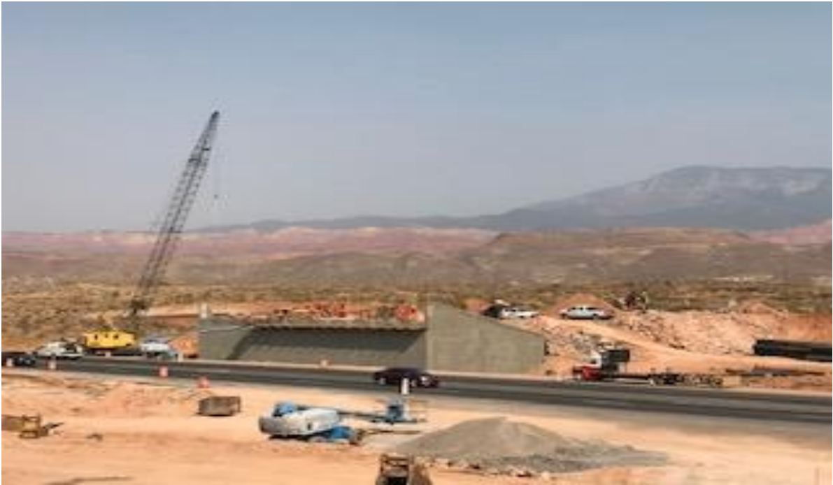
Construction of future overpass at SR-9
